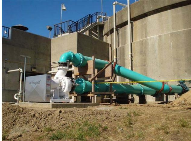
while Digester 2 (gas mixing) generates 68,546 BTU output per KW input daily. This represents a 49.4% increase in overall efficiency of the Digester 1 mixing system vs that of Digester 2.
